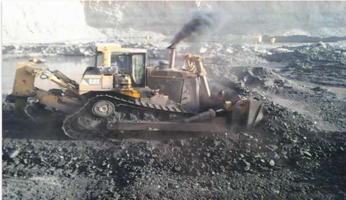
Fig. 6: Mechanical coal removal by bulldozer
